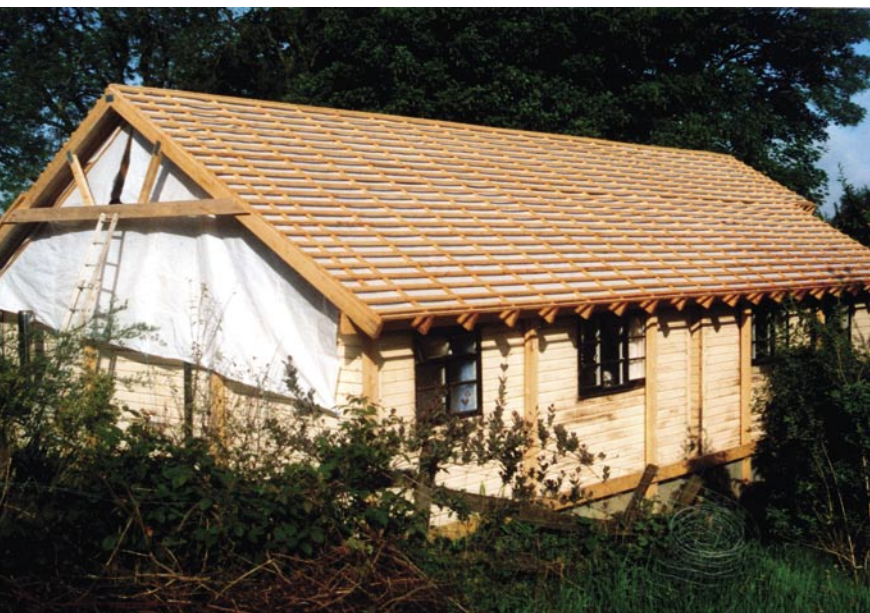
Jerry Clarks homegrown cedar clad home 'The Cabin' under construction
