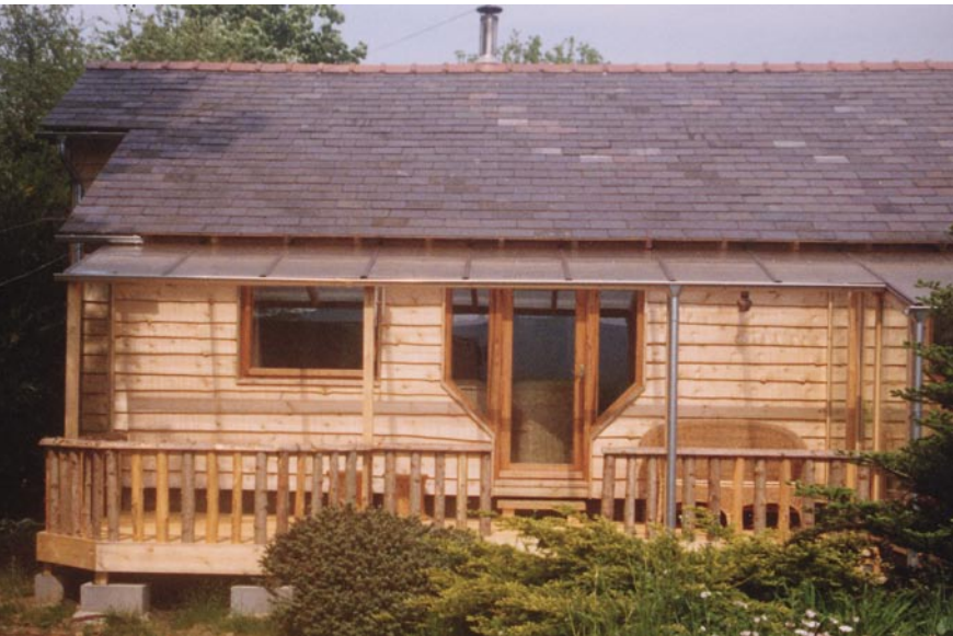
'The Cabin' after completion
