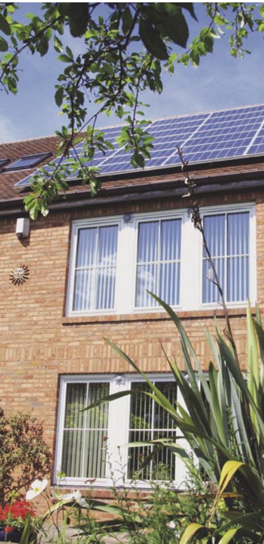
Front elevation of Solaria showing the pv array and large south facing windows
