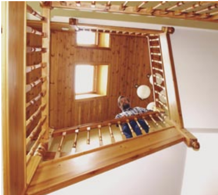
The solar chimney in Solaria proved to be less effective as a cooling device than simple cross ventilation
